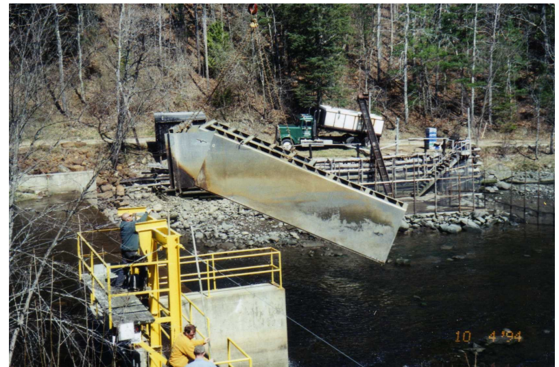
Installing the repaired fish way 2012
