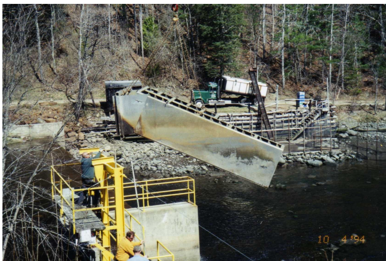
Installing the repaired fish way 2012
